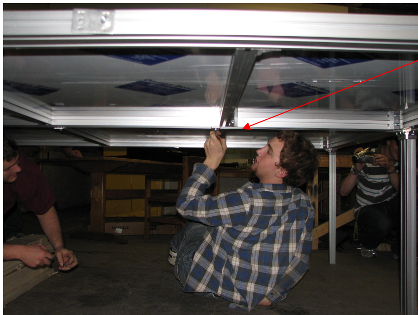
Figure 5 - Attaching Joining Plates on Bottom side of Table Assy
